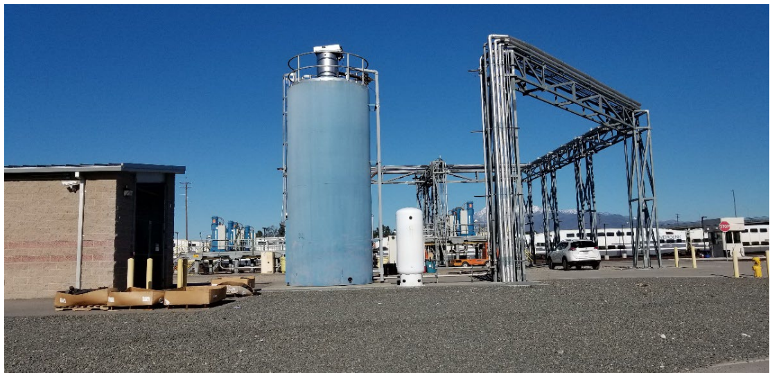
FIGURE 1-H. OVERHEAD PIPED SANDING FROM SAND SILO
