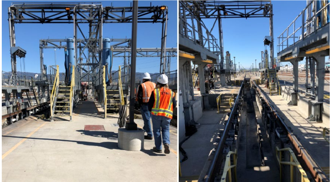
FIGURE 1-G. PLATFORMS AT END OF S&I POSITION
