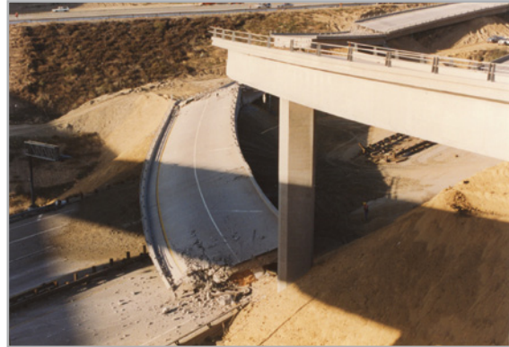
Damage caused by the Northridge earthquake
