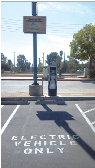
Charging slot at the Sylmar/San Fernando Station
